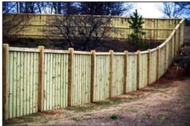
Figure 6-6: Finished Side Facing Exterior
